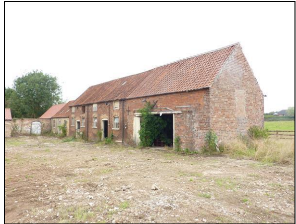
THE EXISTING BARN
