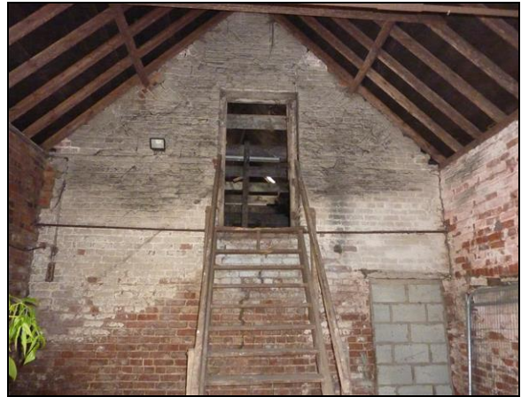
THE EXISTING BARN
