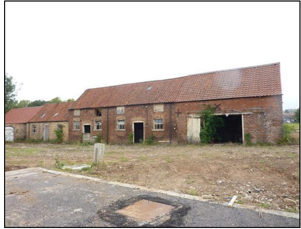
THE EXISTING BARN
