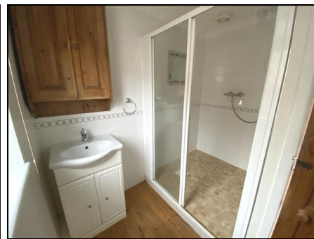
Wet Room Shower Room
